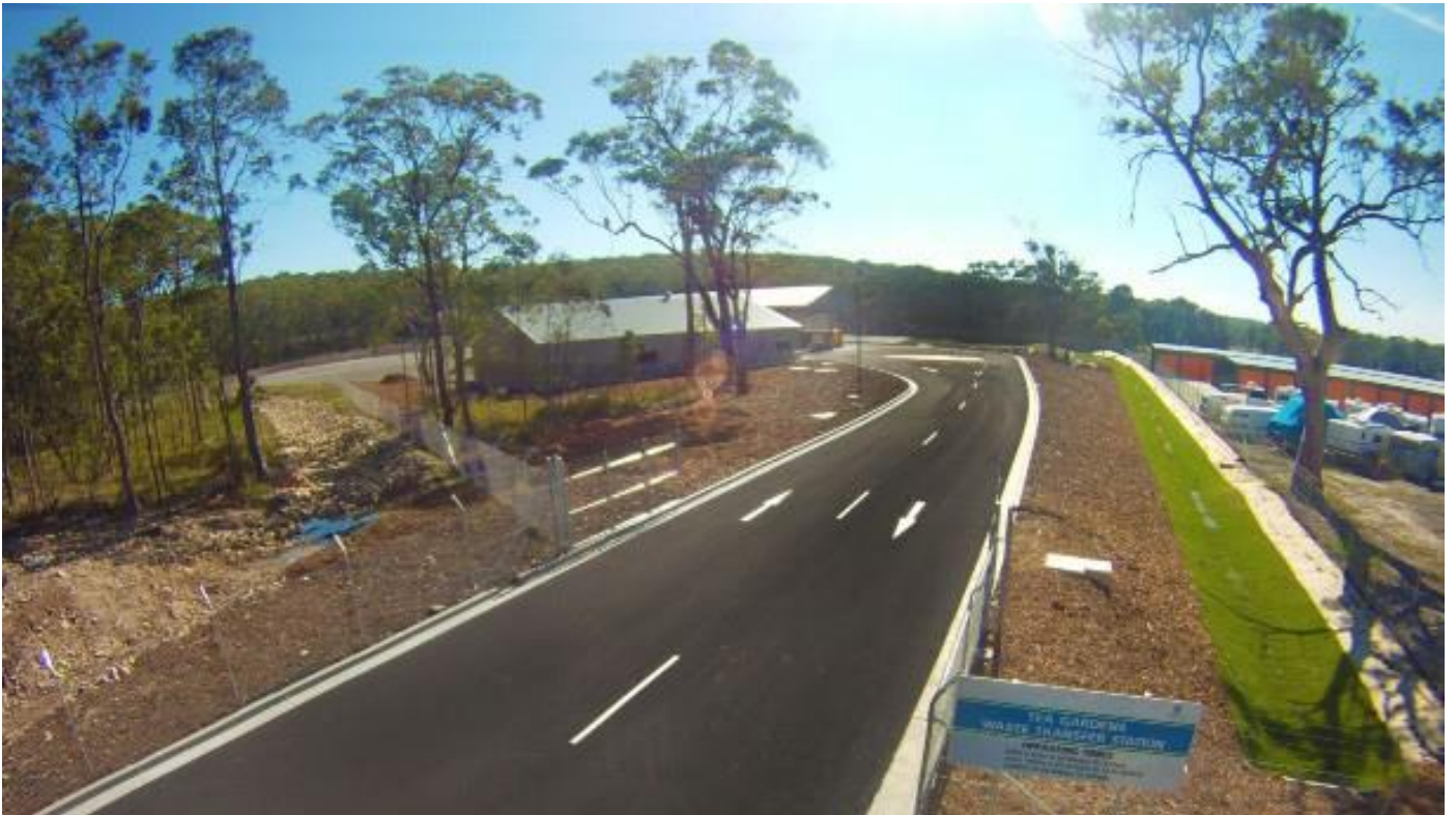
Entrance to the Tea Gardens Waste Transfer Station
