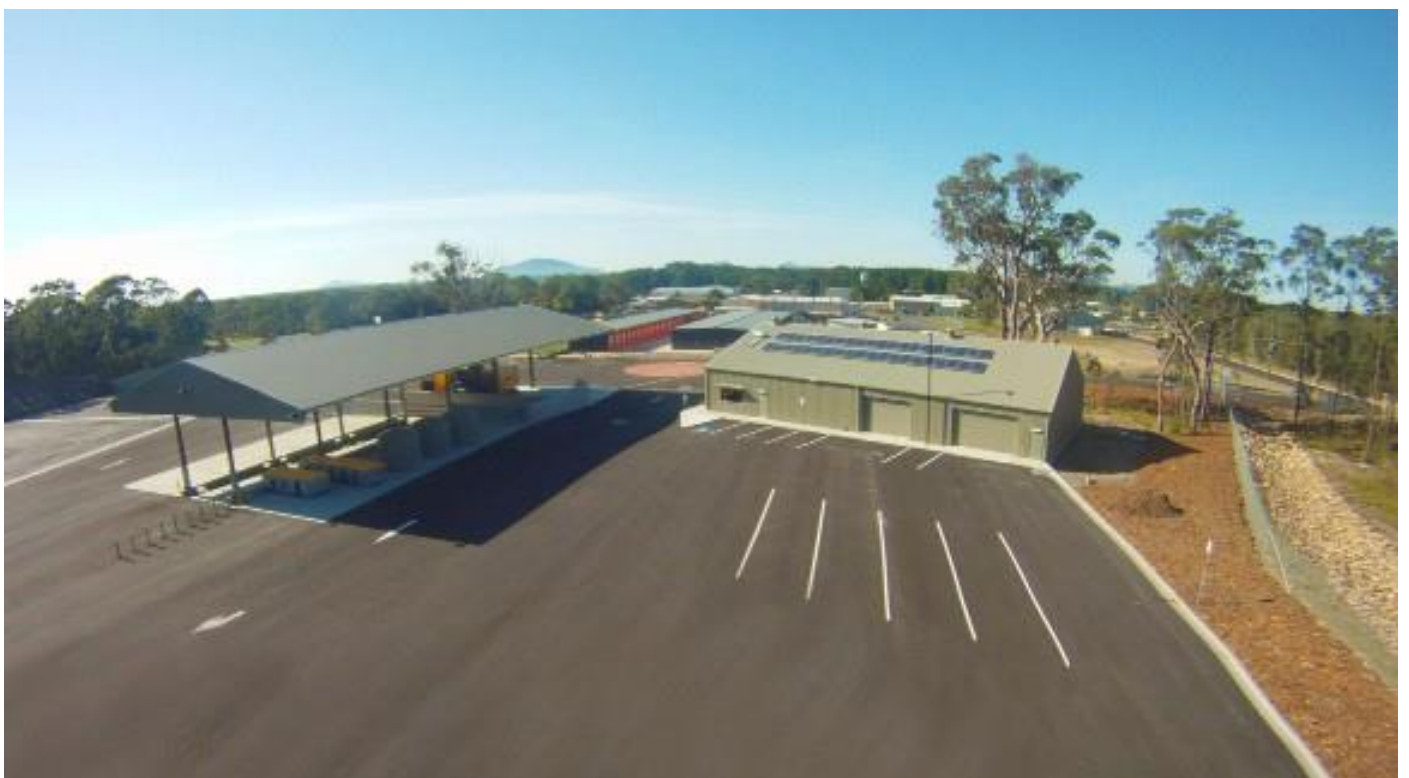
Waste transfer station
